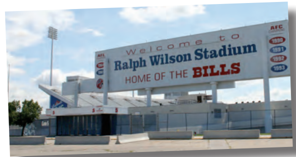
Ralph Wilson Stadium
