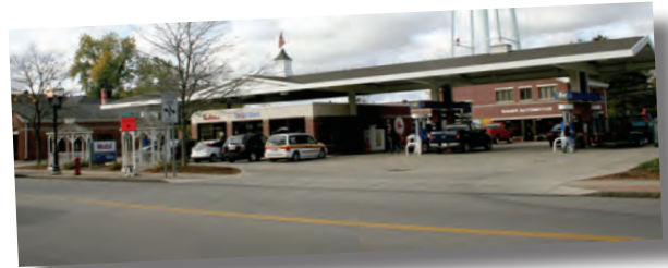
Bauer Service Station
